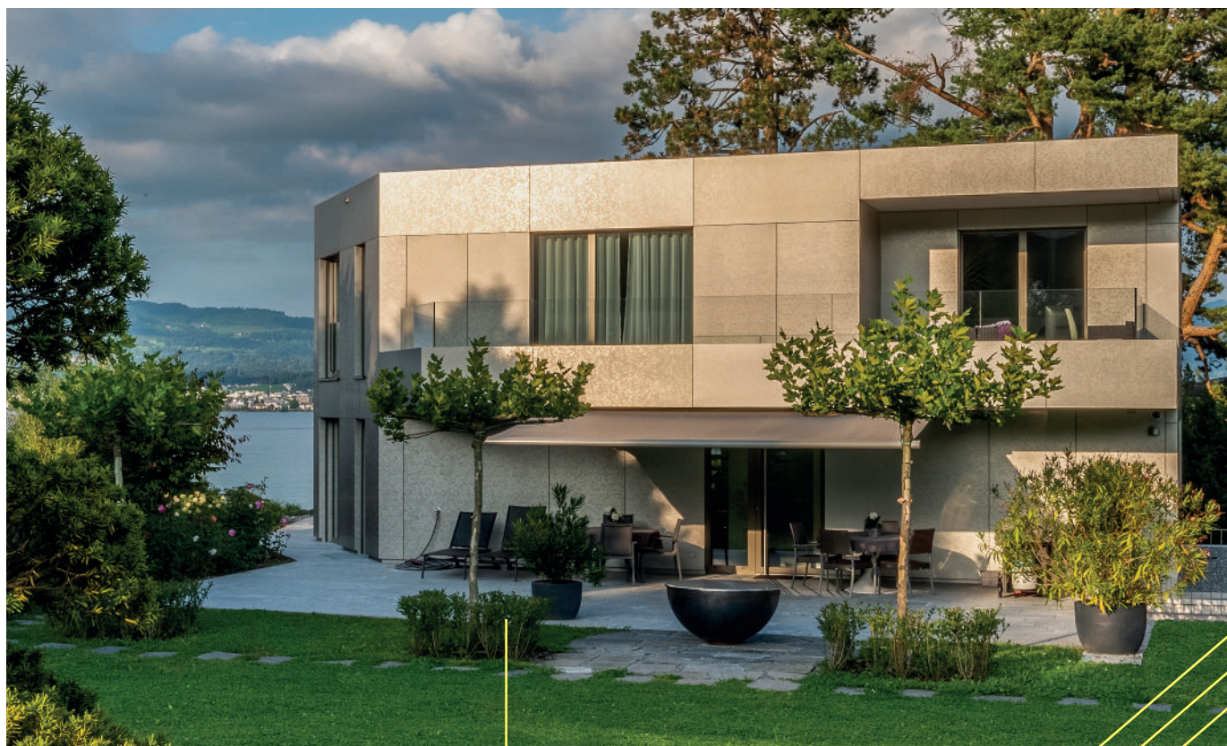
Villa Altendorf, Switzerland Contractplan AG © Allega GmbH
